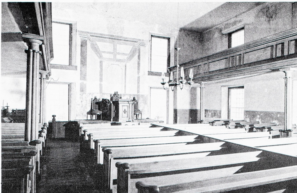
Rustically attractive church interior.
